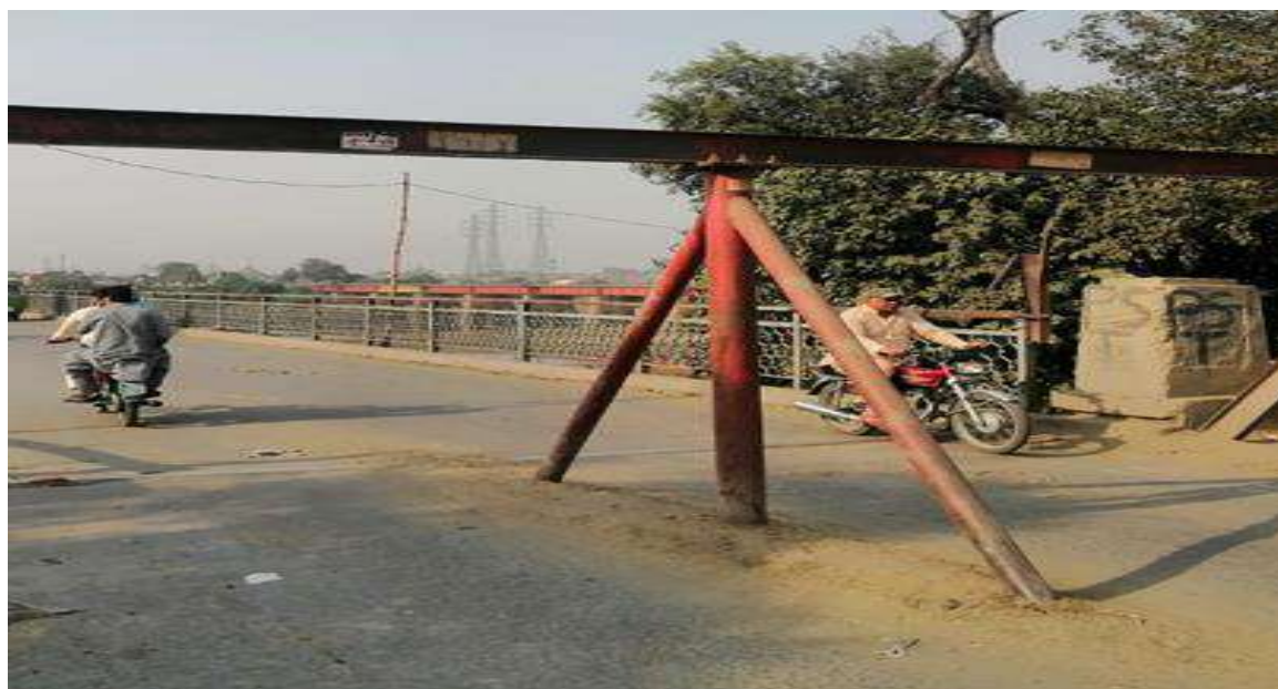
Figure 5-1 Heavy Vehicle Restriction Barrier at entrance and exit
