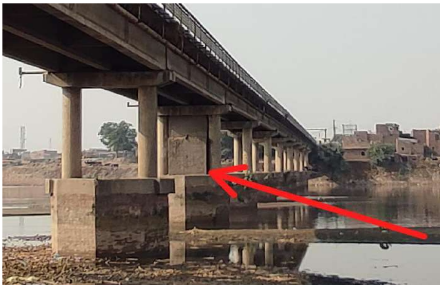
Figure 5-4 Brick wall between the piers
