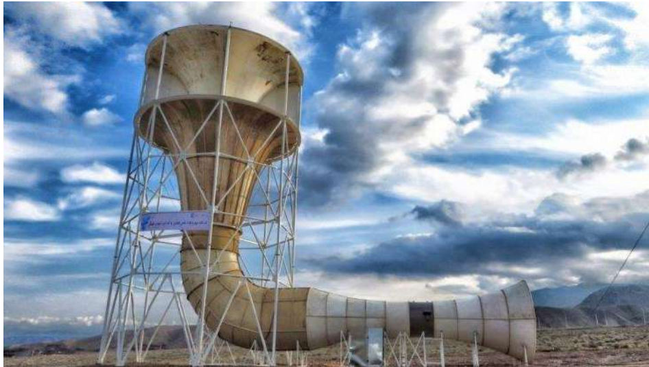
Fig. 1.1.4. Omni-Directional Anemocone
