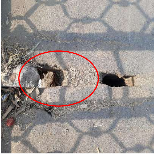
Figure 2.11 Stones on the deck slab
