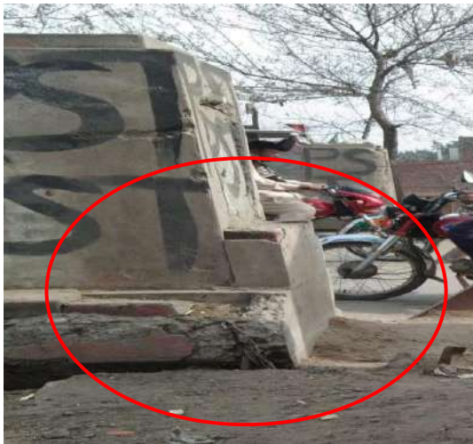
a) Removal of concrete from surface
