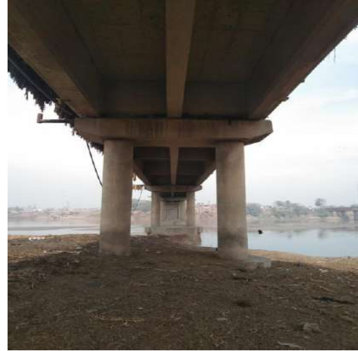
b) Bottom view of Girders and floor beams
