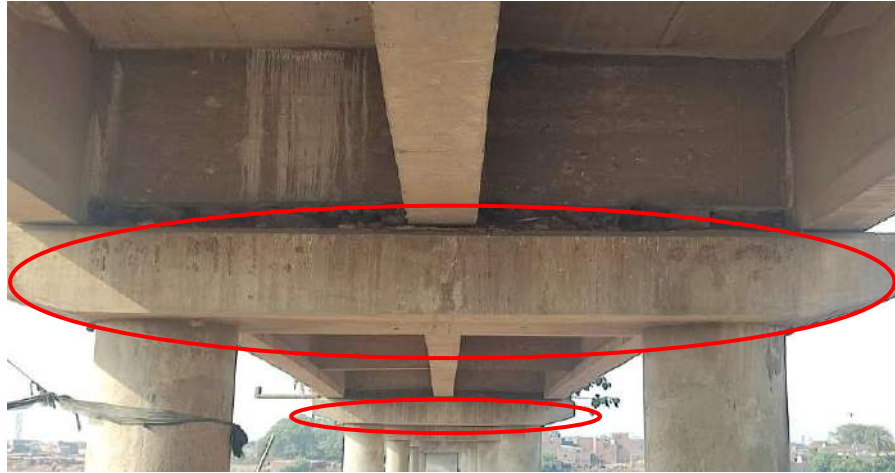
Figure 2.18 Pier Cap Inspection
