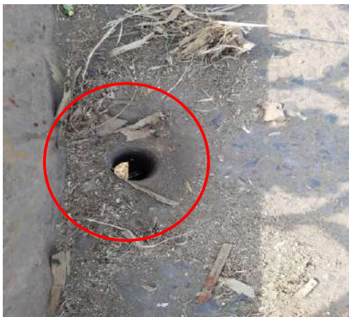
Figure 2.13 Holes drilled on wearing surface
