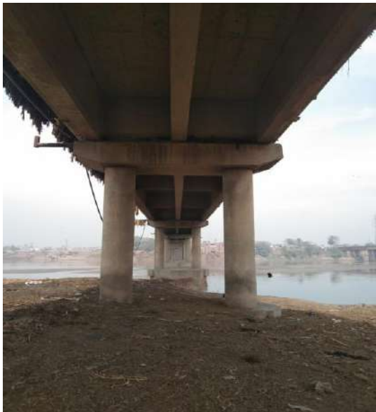
a) Bottom view of piers
