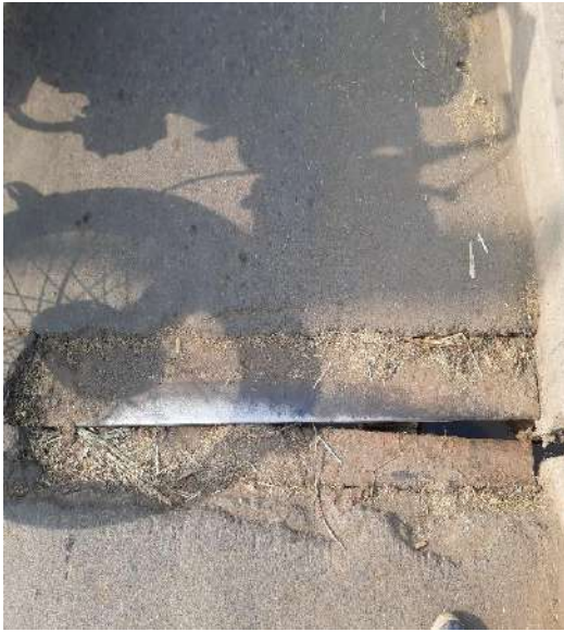
Figure 2.7 Exposed anchorage
