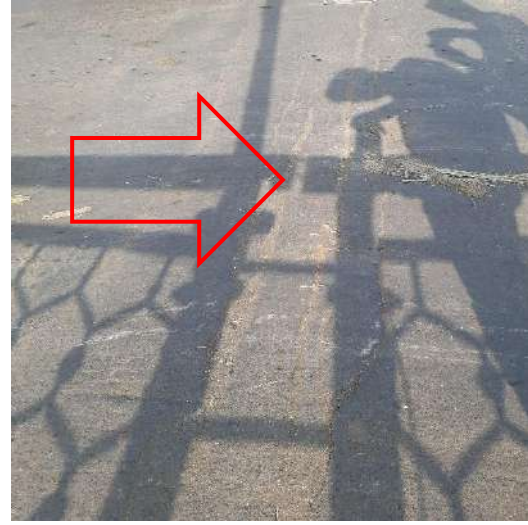
Figure 2.12 Extra Pouring of concrete
