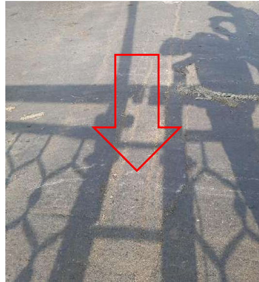
Figure 2.8 Joint filled with concrete
