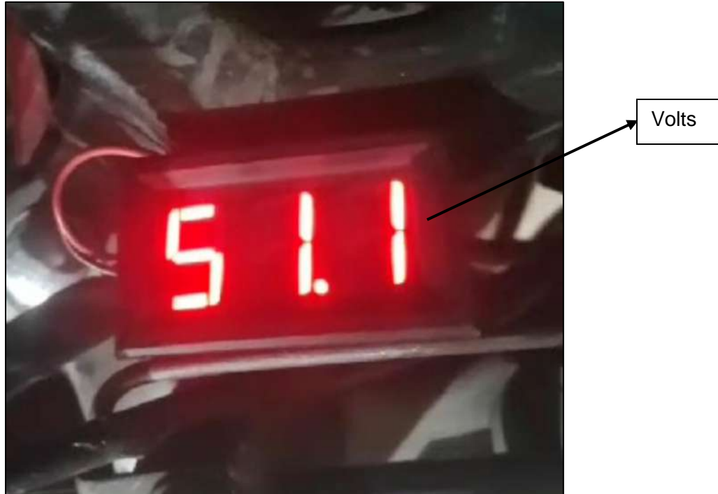
Figure 1. 11: Battery Charging Display
