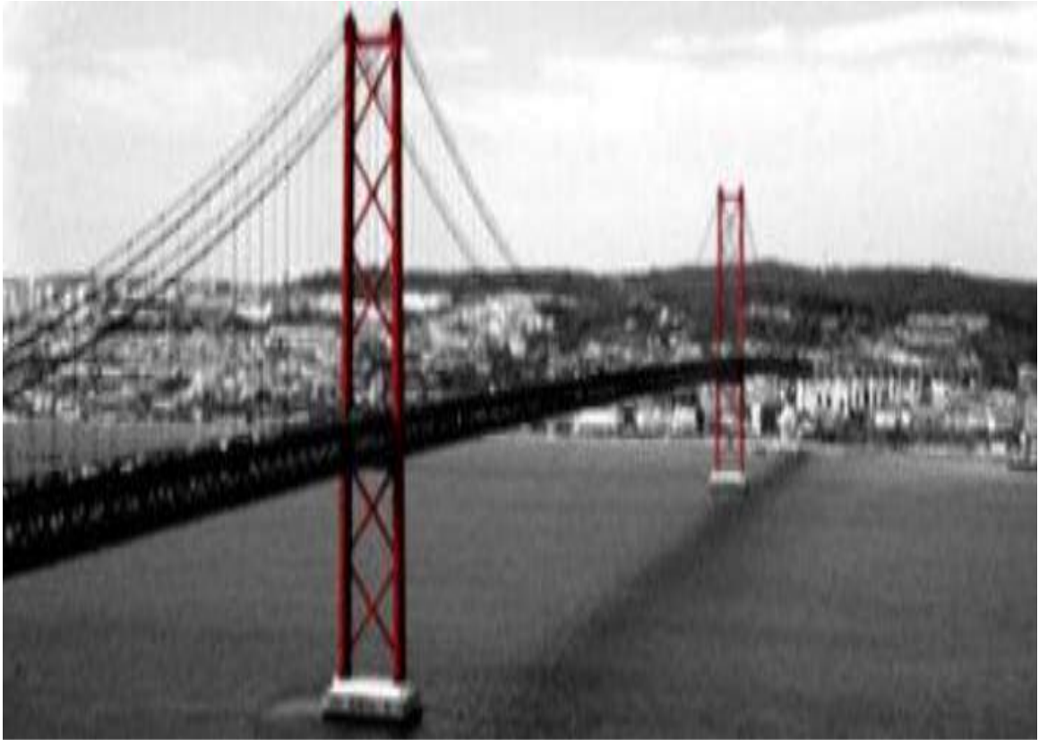
Figure 2.2 Ponte 25 De April
