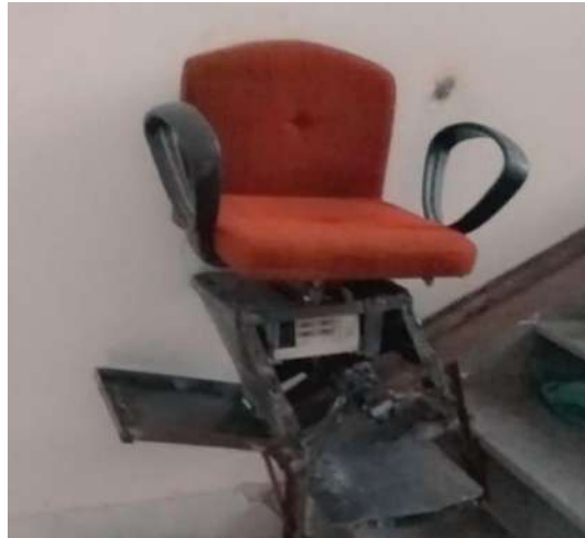
Figure 4.2: “Stairlift” installed at the stairs (new building) Electronic Engineering department of MUET Jamshoro .
