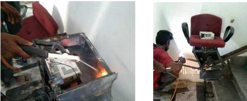
Figure 3.22: Skeleton coverage using iron sheets through welding
