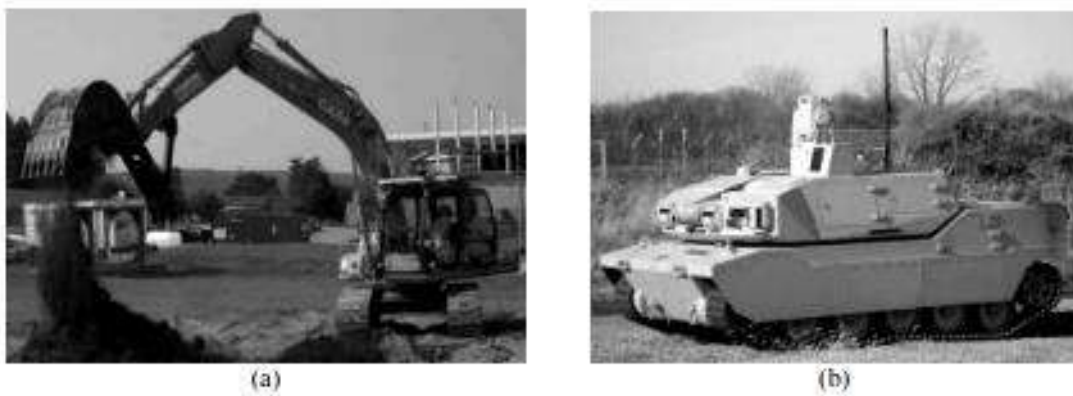
Figure 2 REMOTE CONTROLLED VEHICLE (a) Excavator (b) Unmanned ground vehicle
