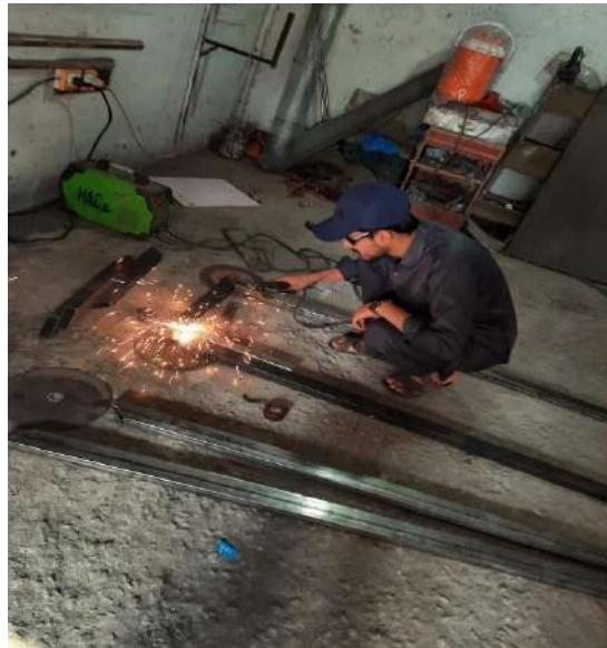
Figure 3-21: Frame Welding short
