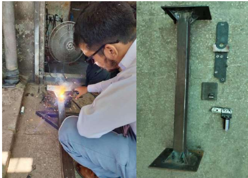
Figure 3.13: Parts Fabricated by Welding
