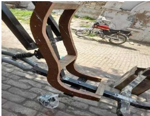
Figure 3-34: Building the Cradle
