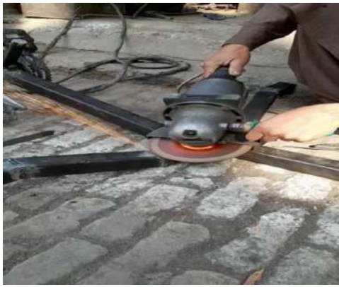
Figure 3-32: Grinding of welding parts
