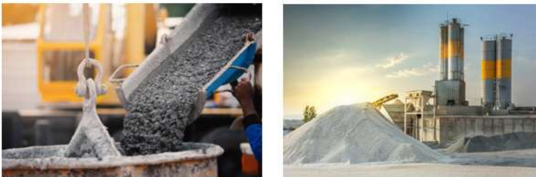
Figure 1.1: Concrete Mixing Station
