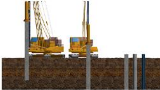
Figure 6: Driven of Piles
