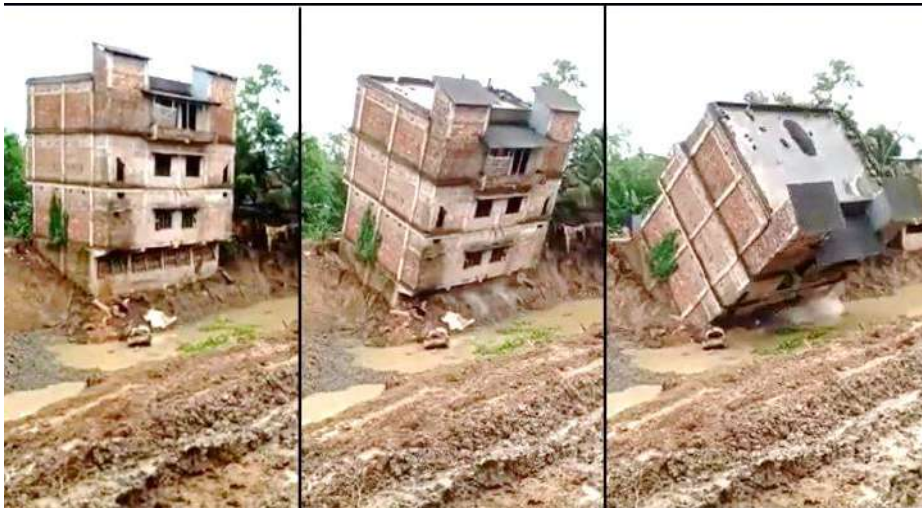
Figure 2.1. Foundation Failure Due to Presence of Untreated High Plastic Clays
