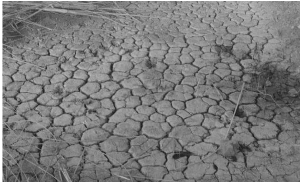
Figure 1: Expansive Soil of Nandipur Pakistan with ground cracks
