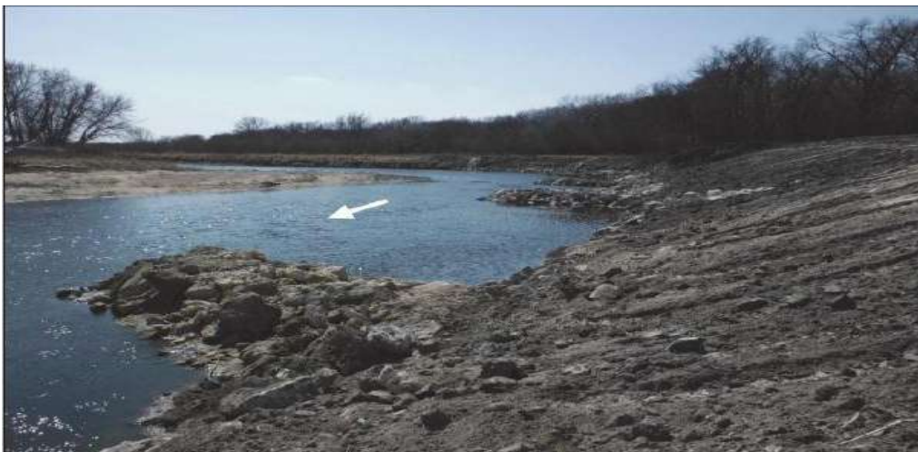
Figure 2.4: Spur dikes for stabilizing purpose
