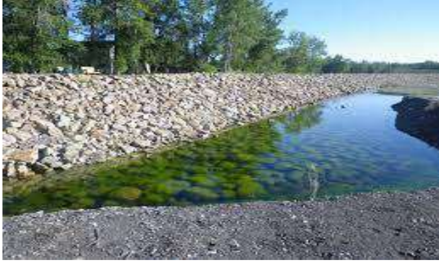
Figure 2.9: Riverbed armoring
