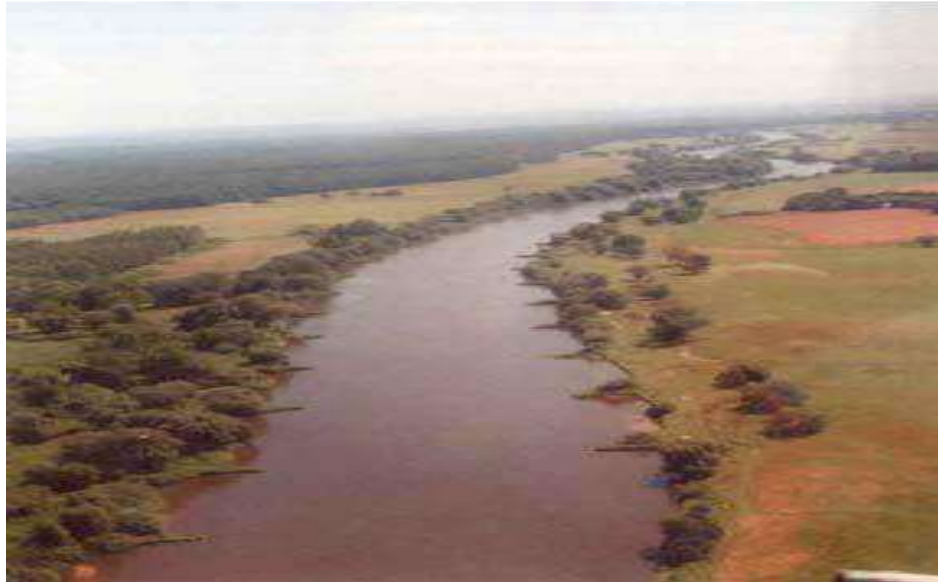
Figure 1.1: Spur dike fields; Odra River in Poland
