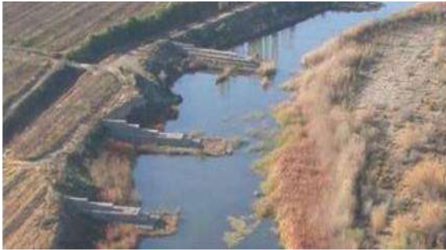
Figure 2.8: Spur dike protection at Gamka River, South Africa
