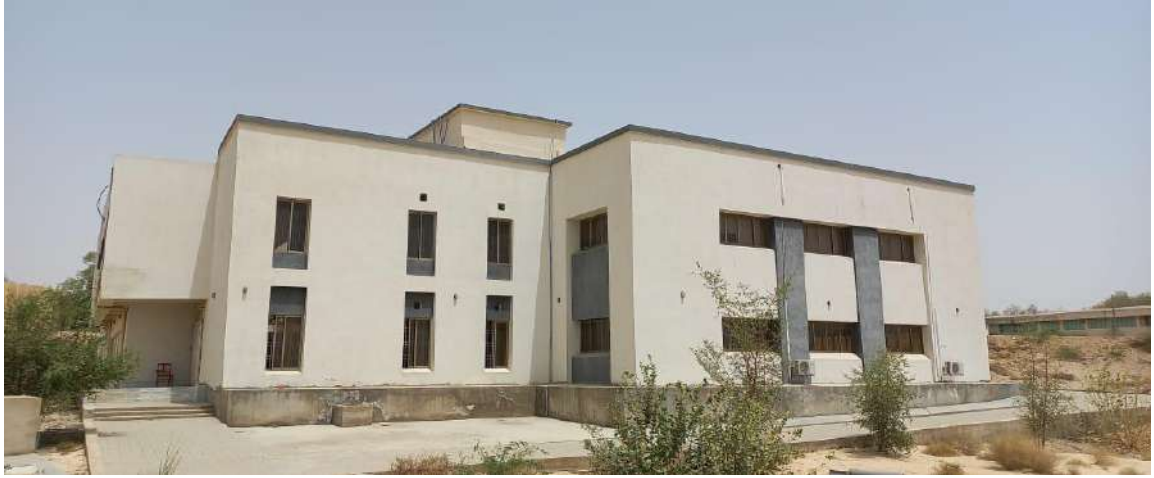
Fig 1.3: Front view of the building
