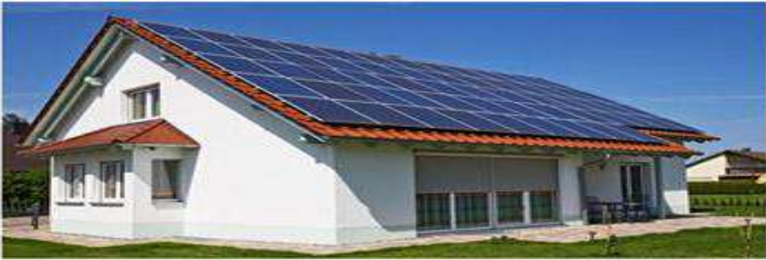
Figure 2.2 Residential Roof-Top PV 1
