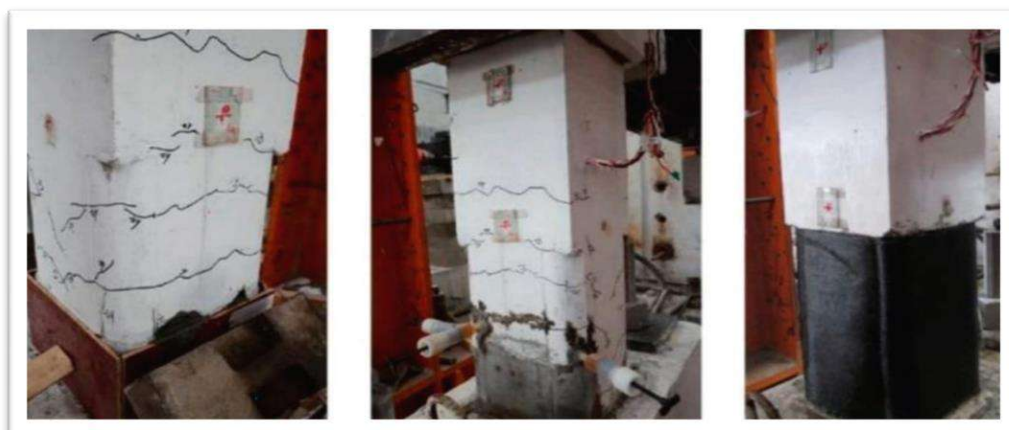
Figure 2.18 Testing of Column
