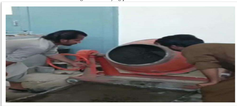
Figure 3.13 Concrete mixing on mixer
