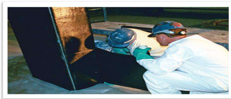
Figure 2.3 Column Axial Enhancement with FRP sheets
