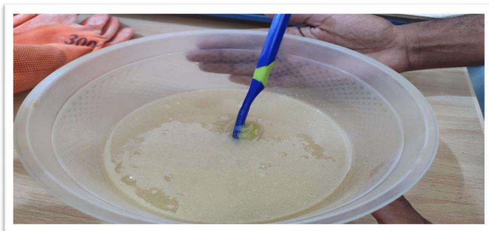
Figure 3.27 Mixing of Epoxy
