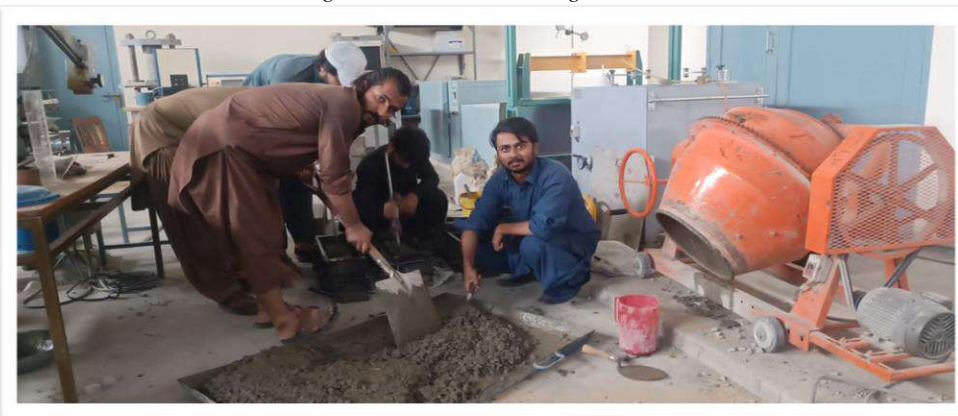
Figure 3.14 Manual mixing of concrete
