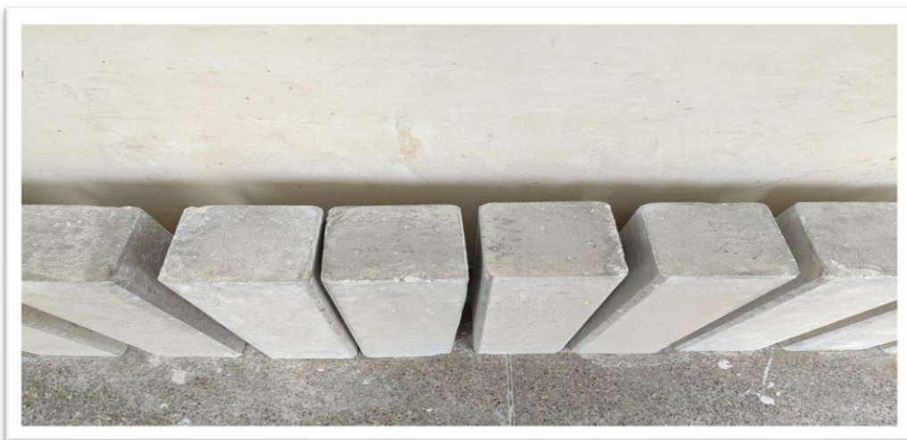
Figure 3.24 After surface finishing
