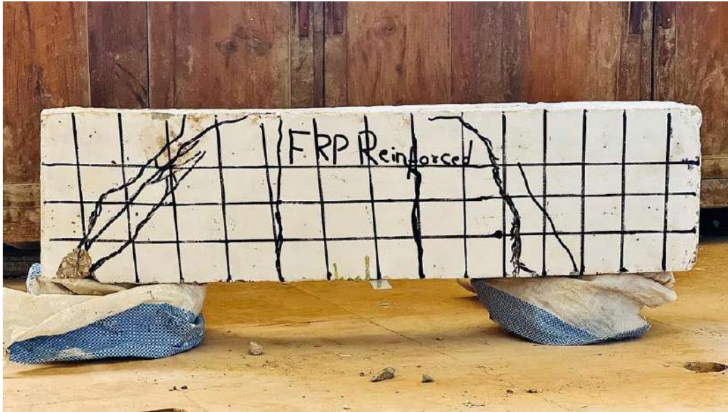
Figure 4. 20: Cracks Pattern in FRP Beam 1
