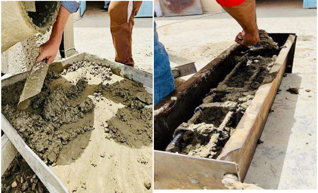
Figure 4.9: Placement of Concrete.
