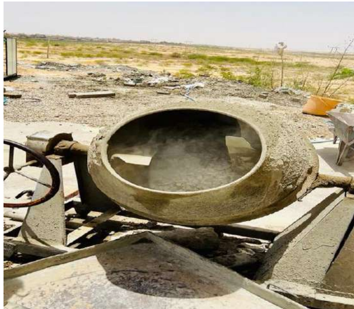
Figure 4.8: Mixing of Concrete in Mixer
