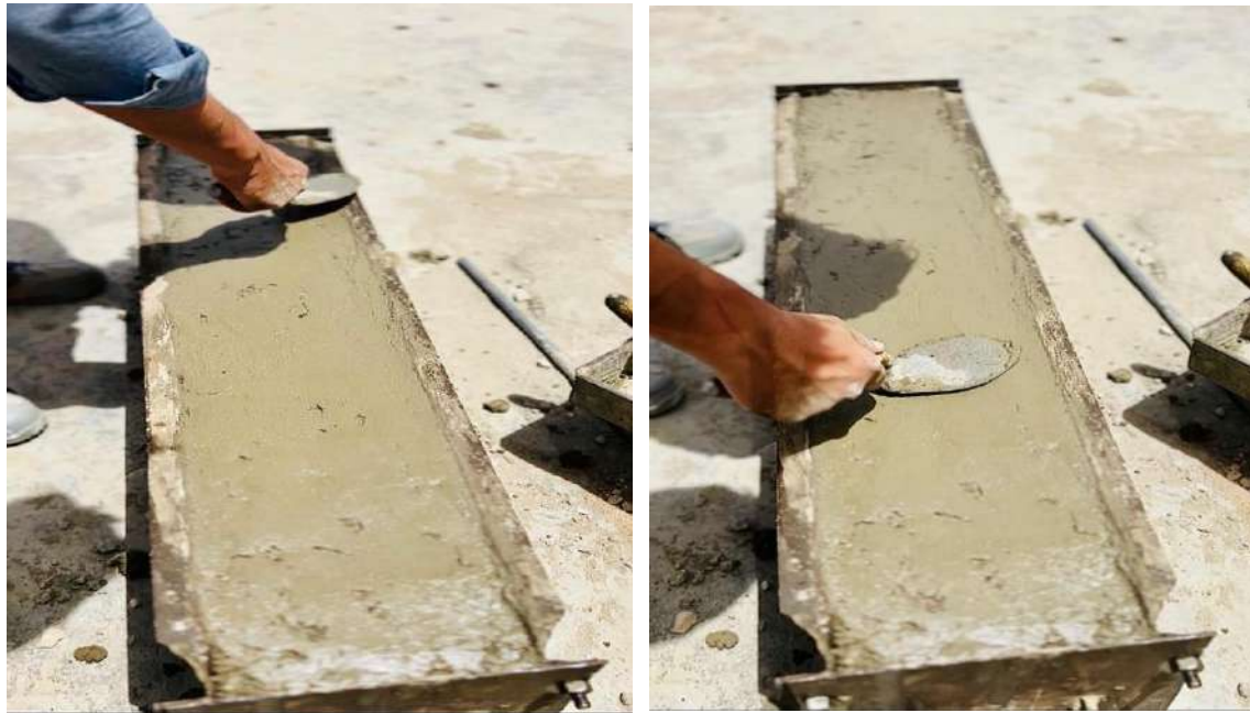
Figure 4.11: Finishing of Concrete beam
