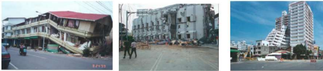
Figure 5: Building damages in 9-21 Chi-Chi earthquake (Tsai et al., 2000)
