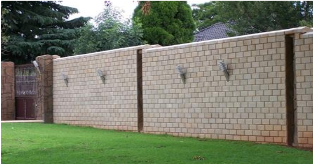
Figure 2.3 Boundary wall with interlocking block
