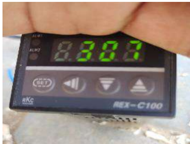
Figure 4.25. Exhaust Gas Temperature Measuring
