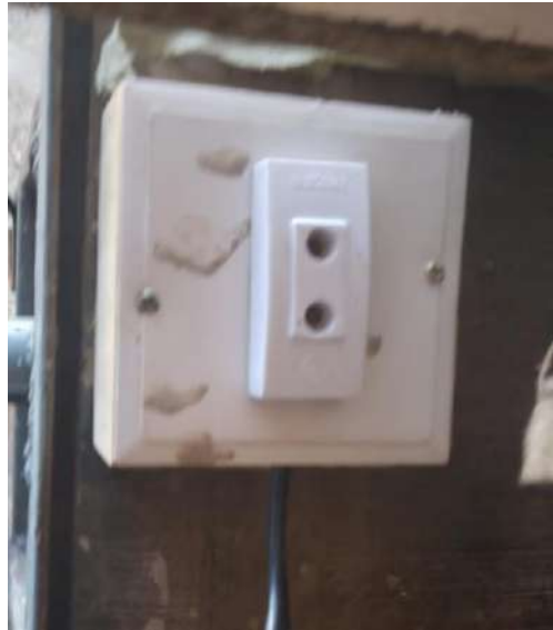
Fig 4.21: Installation of the board of generator output [10-04-23]
