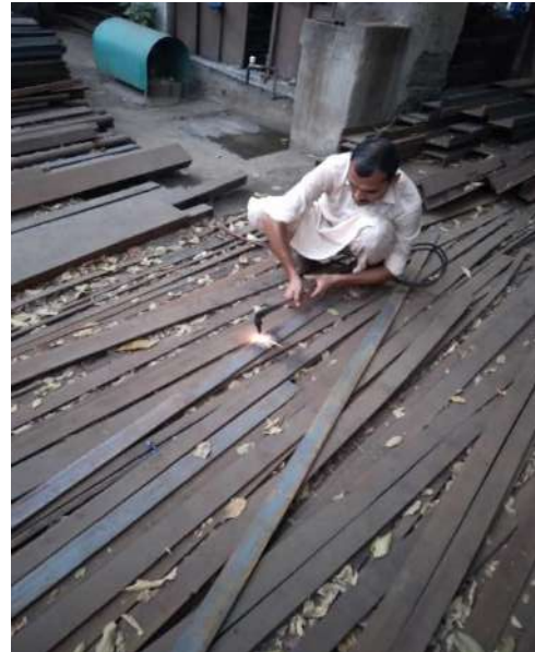
Figure 3-7: Hard iron cutting by gas cutter [22-9-22]
