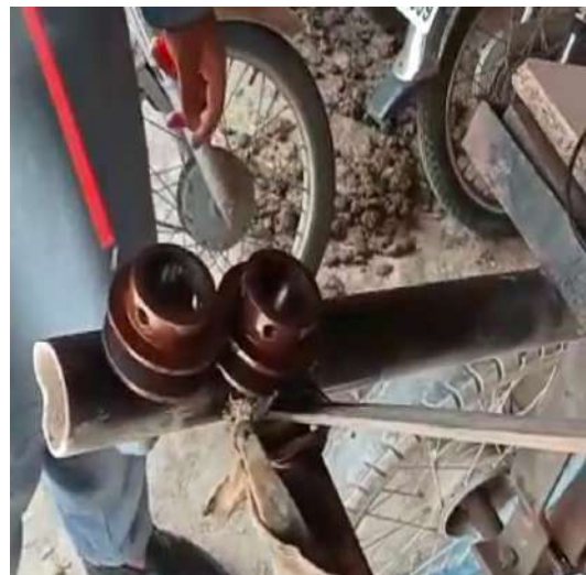
Fig 4.26: Another view of Spray on rusted pulleys [12-04-23]
