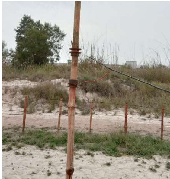
Fig 4.28: connection of generator & pulleys [12-04-23]
