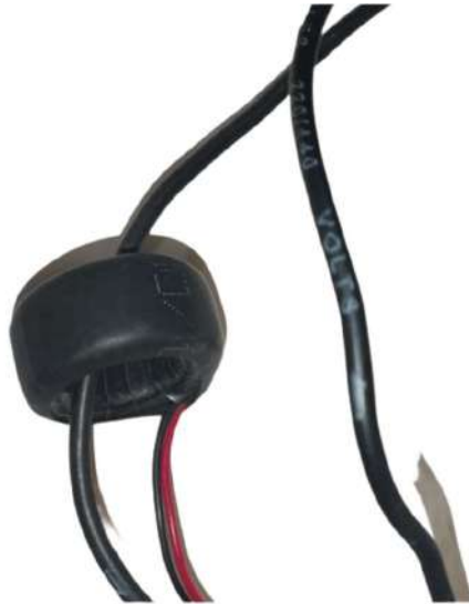
Figure 63: Live Wire Through CT connected to Load.
