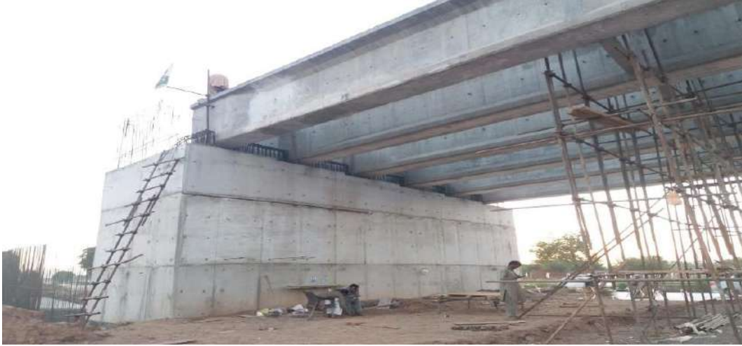
Figure 1-0-1: Rawal Chowk Bridge Islamabad
