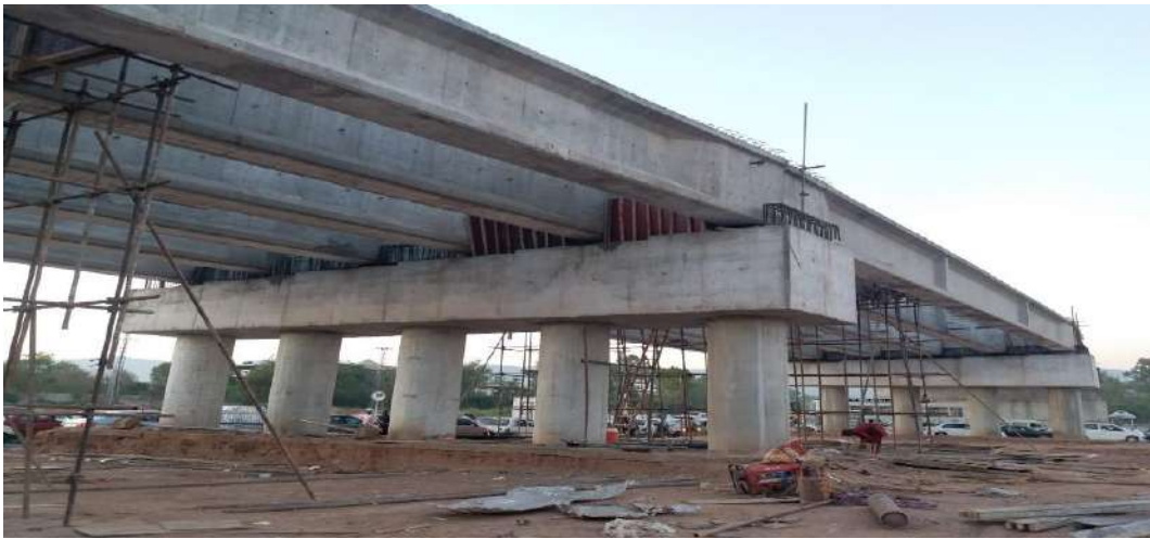
Figure 1-0-2: Rawal Chowk Bridge Islamabad
