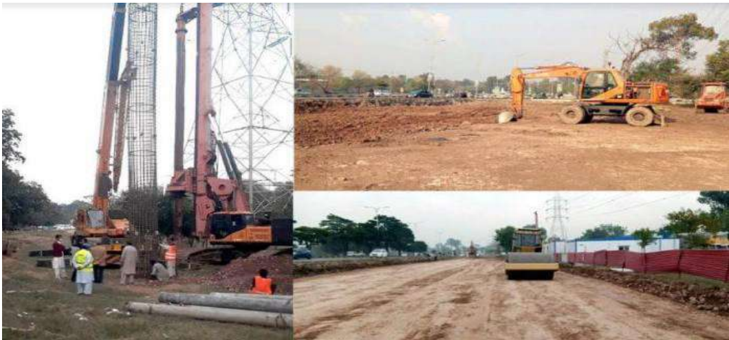
Figure 1-0-3: View Of Under Construction Rawal Chowk Flyover
