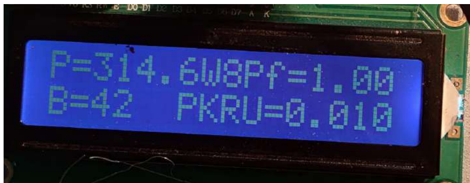
Figure 4.22: Parameters display of energy meter
