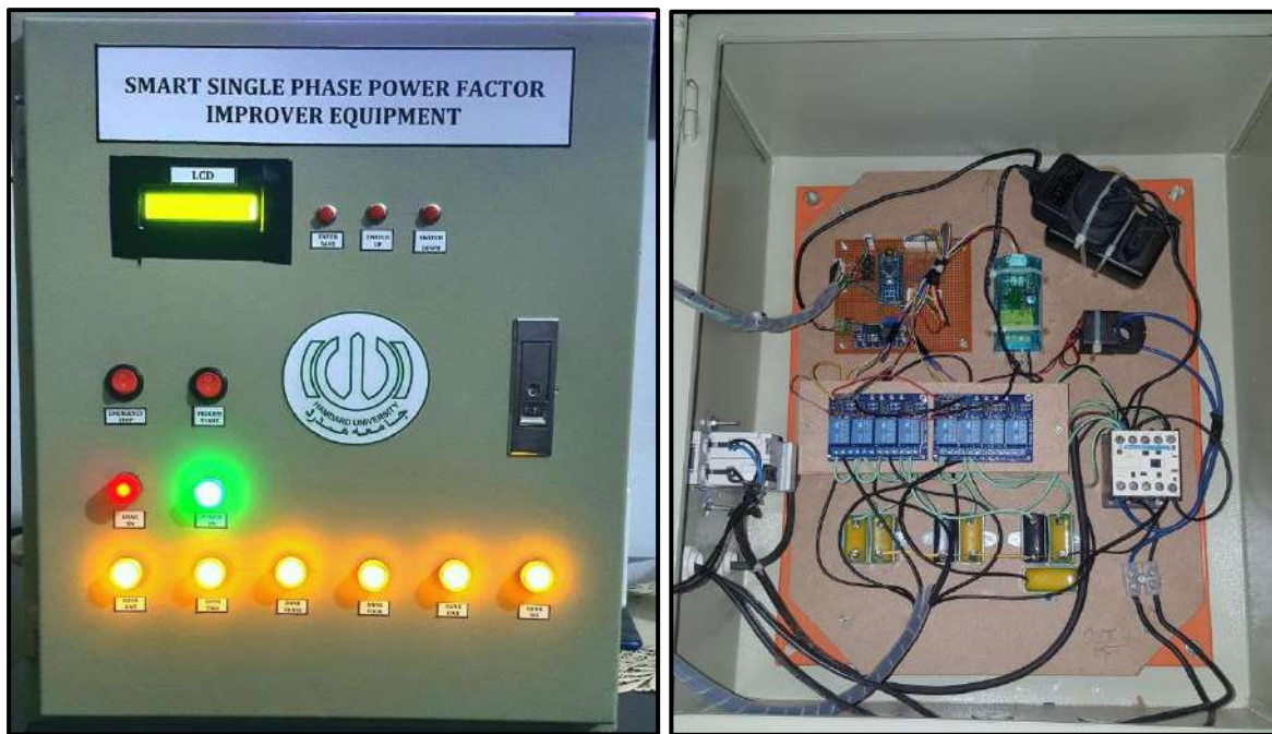
Figure 4.25: The Completed PF Correcting Equipment
