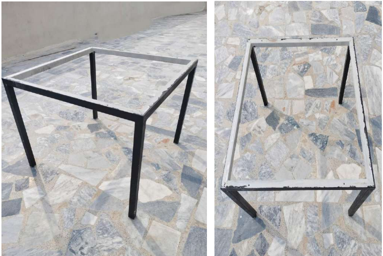
Figure 7-1: Fabrication of Lower Frame
