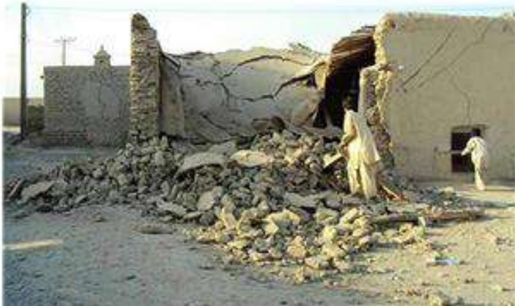
Figure 3.5 Aftermath of Harnai Earthquake 2021
