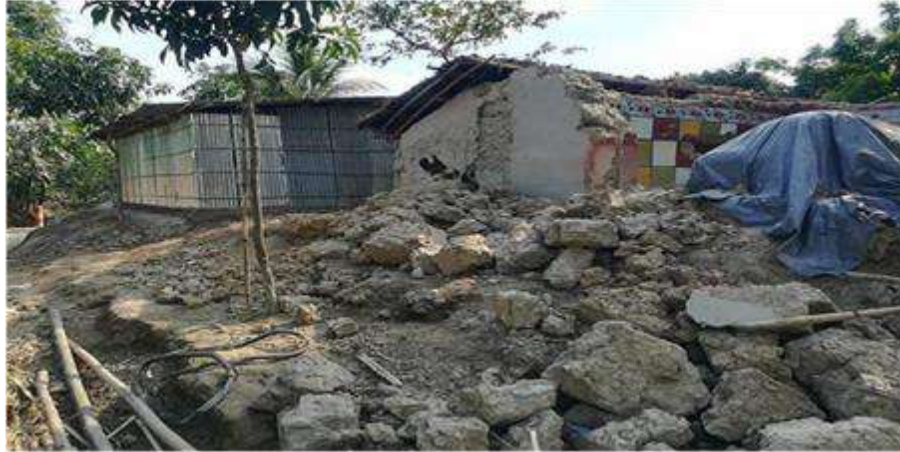
Figure 3.3 Failure of adobe structure after earth quake in Ziarat in 2021
