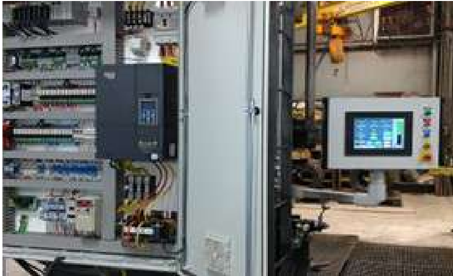
Figure 1.4: PLC based monitoring and control system
