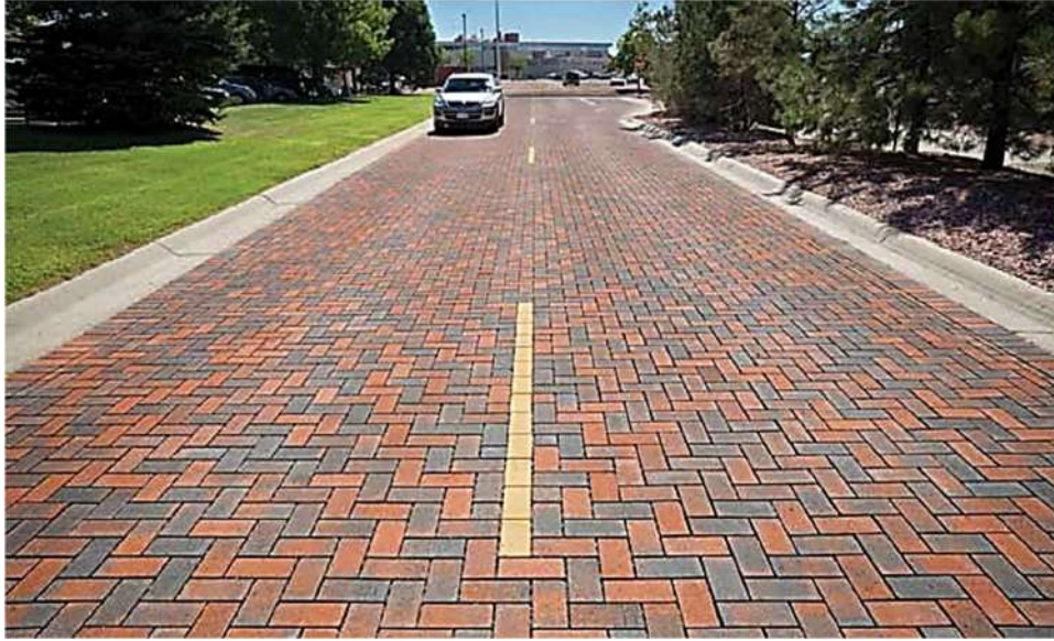
Figure 2. 7: Permeable concrete pavers for road surfacing (paving stone pavement) (Maty, 2022)
