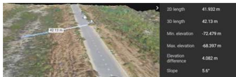
FIGURE 6.16: Elevation between the road and ditch
